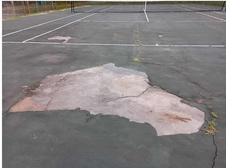
Pictures showing significant delamination of the surface of Courts 2 and 3 which will be addressed in the proposed repairs
