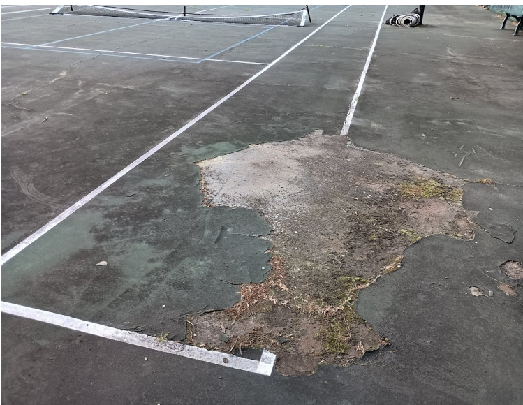
Pictures showing significant delamination of the surface of Courts 2 and 3 which will be addressed in the proposed repairs
