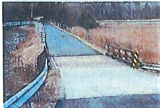
01.3: QUEENS LAKE DRIVE BRIDGE CROSSES THE SPILLWAY
