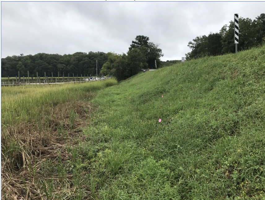
07 – Looking SE Downstream Embankment
