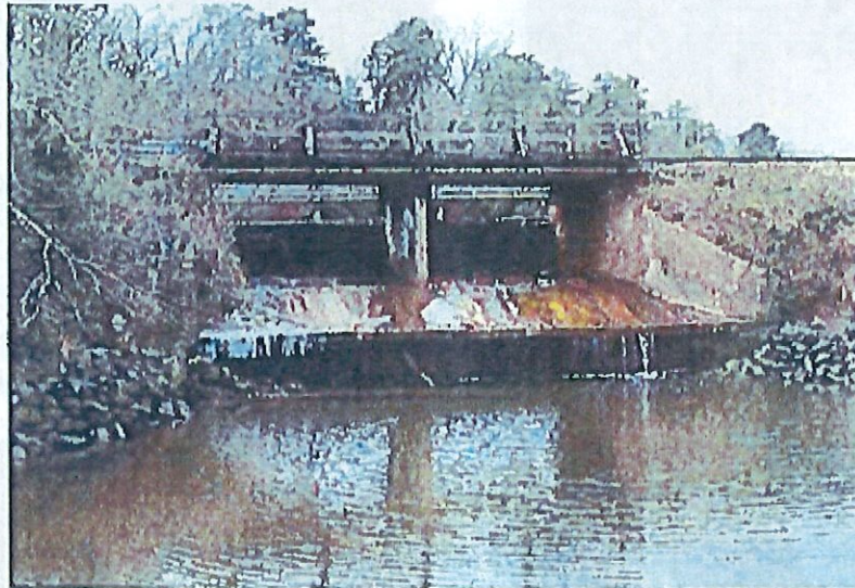
01.1: OVERALL PHOTO – SPILLWAY ON THE NORTH FACE
