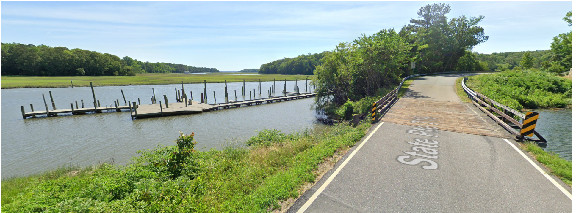
09 – Spillway Inflow & Outfall Looking Downstream of Queens Creek (May 2019)
