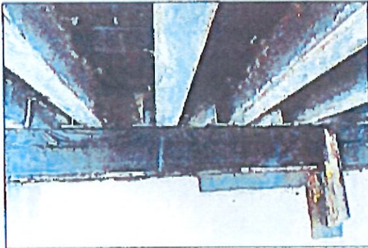
01.8: HEAVY TIMBERS CAP THE CONCRETE ABUTMENTS TO SUPPORT BRIDGE STRUCTURE
