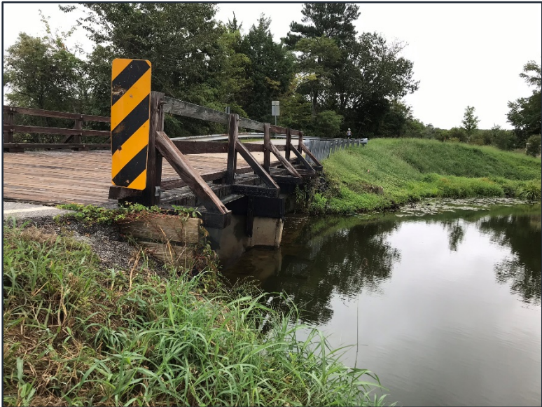
Picture 2.2 – Queens Lake Spillway Inflow
