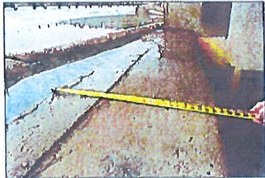
01.9: THE CONCRETE STRUCTURE APPEARS TO HAVE BEEN CONSTRUCTED IN VARIOUS SECTIONS
