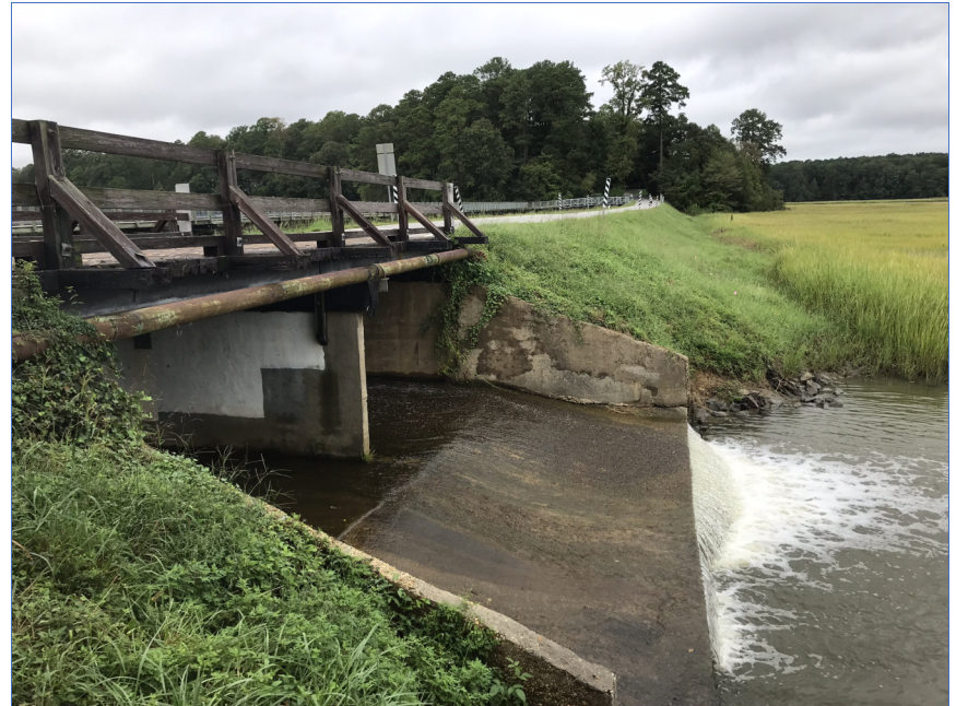
06 – Looking NW Outfall & Embankment
