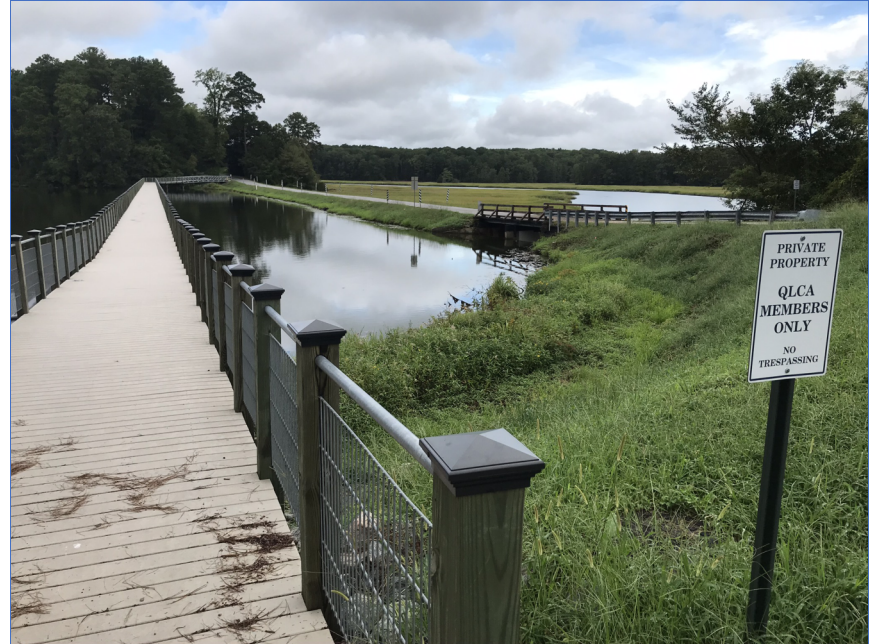
02 – Looking NE Across Embankment
