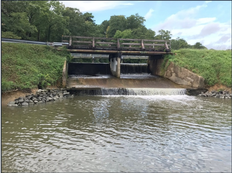
Picture 2.1 – Queens Lake Dam Spillway Outfall
