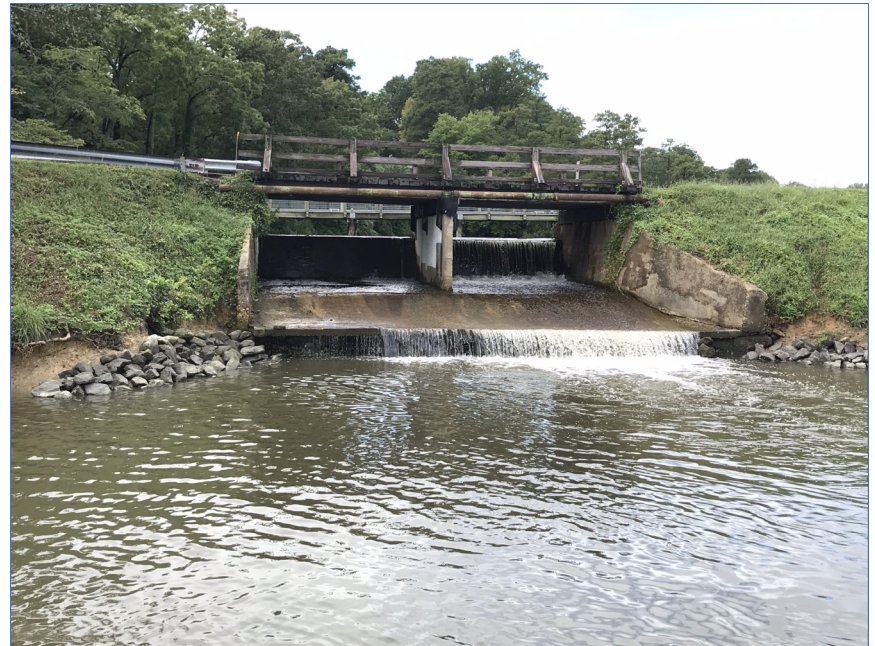
04 – Looking at Spillway Outfall
