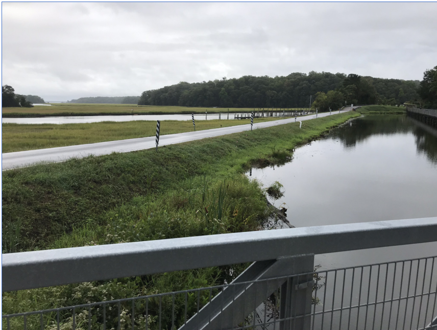
03 – Looking SE Across Embankment
